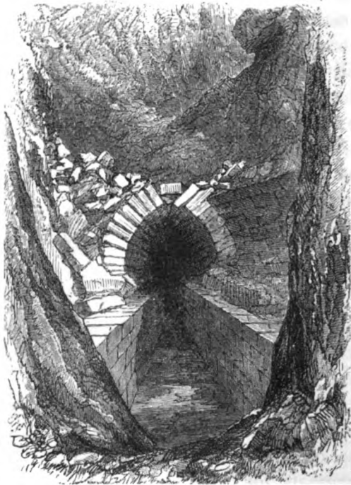
Arched drain (South-East Palace, Nimrud).
