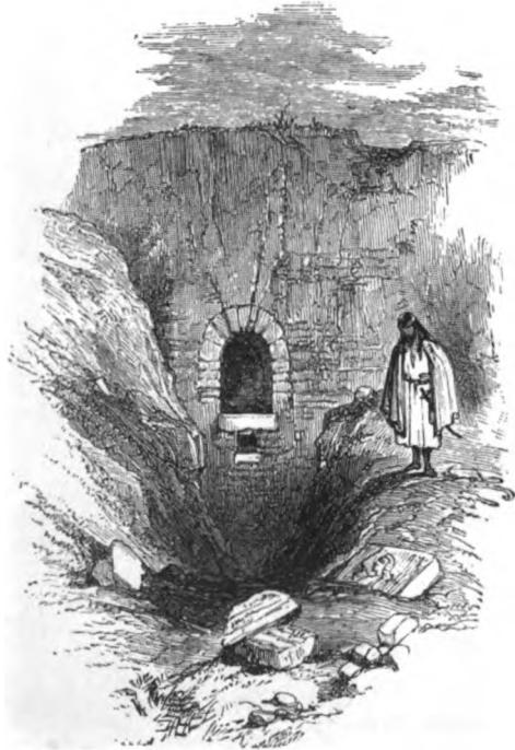
Arched drain (North-West Palace, Nimrud).
