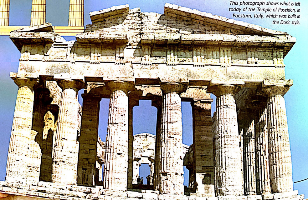
The architrave (lowest part of the entablature)
